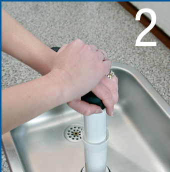
2 Use the weight of your body to press hard onto the piston. Press a few times..
